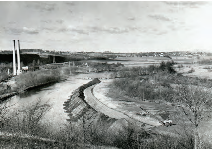
A dragline moved sediment from the river's banks into the channel. Harold Amster. Used with permission of the Spring Ford Area Historical Society.
