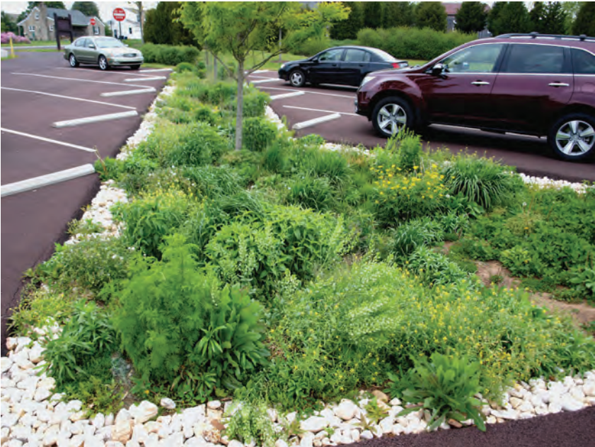
2012 photo showing a rain garden in the parking lot of Black Rock Sanctuary. Sustainable stormwater best management practices were incorporated into the development of the Black Rock Sanctuary. John Mikowychok. Used with permission.
