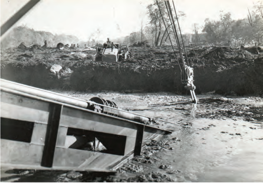
Sediments that had accumulated in the floodplain were bulldozed into the river so the dredges could move them into the impounding basins. Harold Amster. Used with permission of the Spring Ford Area Historical Society.
