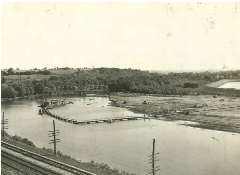
The “Schuylkill” pumping into the Sanatoga Basin in 1949. This image was included in the Final Report of the Schuylkill River Project Engineers . Used with permission of the Commonwealth of Pennsylvania, Department of Environmental Protection.
