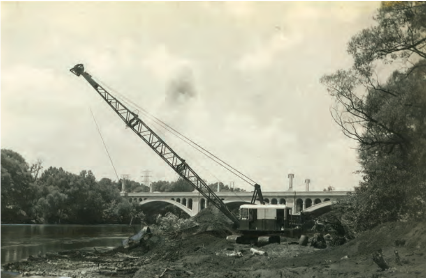
Clearing coal sediments from the Schuylkill's banks near Reading. This image was included in the Final Report of the Schuylkill River Project Engineers . Used with Permission of the Commonwealth of Pennsylvania, Department of Environmental Protection.
