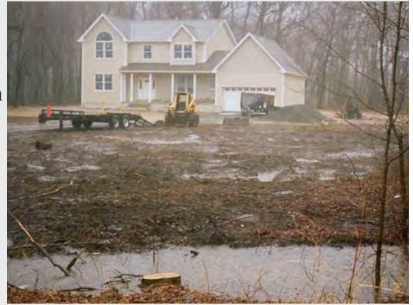
House under construction, Hamilton, Township, NJ. Photo: F. Stine
