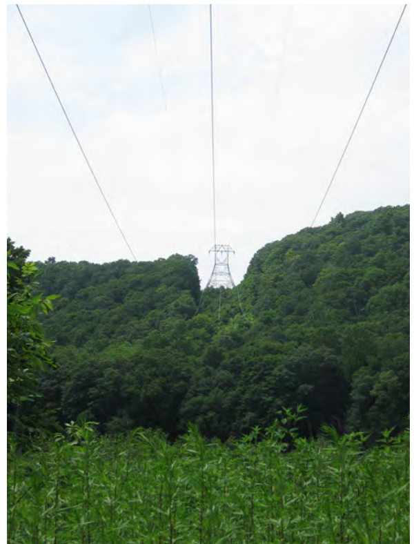
Looking West from Warren Co., NJ, at the current 230kV line on 100’ tall towers. Photo: F. Stine
