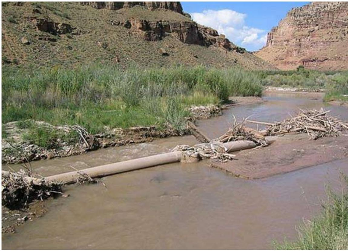
Photo from Fogg and Hadley (2007) of an exposed pipeline crossing an unnamed western US river. Here, lateral migration of a stream channel during high water excavated a section of pipeline under a floodplain that was several feet shallower than at the original stream crossing.
