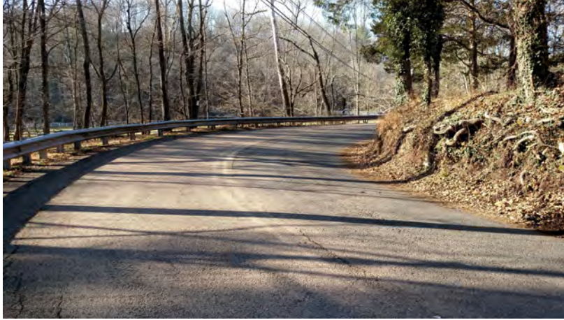
Figure 7 Westbound view of the curve on Headquarters Road located 250 feet east of the intersection with Sheephole Road, the site of 5 crashes within the reporting period
