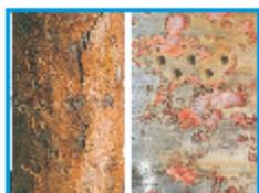
Corroded and pitted casing (Shutterstock). Steel and cement subjected to harsh, corrosive, downhole conditions can degrade in a matter of years, thereby resulting in an explosive, contaminant, and health risk to nearby landowners.
