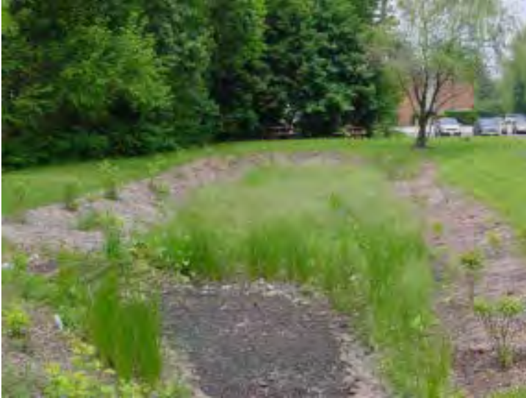
Naturalization of a detention basin and the installation of an infiltration trench (see area of stone).
