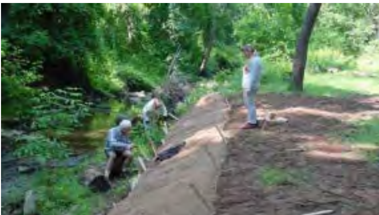
Coir matting installed over a re-graded streambank (Note: Wooden stakes not yet installed completely).
