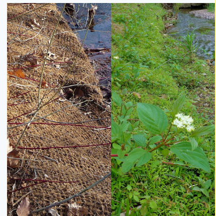
Bioengineering material installed (L); With plant growth (R). J. Nystedt
