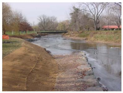
Photo point depicting site after implementation of restoration project that included re-grading and the installation of coir matting and rock vanes. Note footbridge and pavilion in background.
