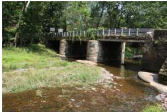
McMullan and Associates Structural Engineers of Vienna, Virginia, has inspected the Headquarters Road Bridge and has determined that this bridge, which is recognized as a historic structure, can be rehabilitated and continue to be a useful element in the county road system. Rehabilitation work would include repairing the existing stone masonry piers and abutments, and improving the existing scour counter measures, using approved materials and techniques. A new one-lane deck would be installed.
