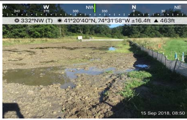
Photograph 6: Vegetation growth observed in W-3 (Huguenot)
