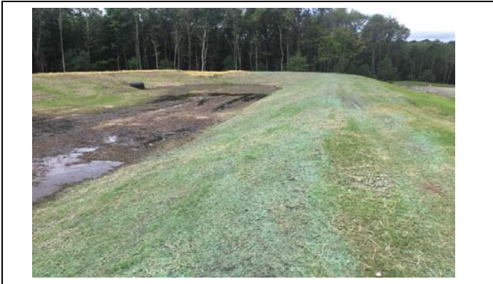
Photograph 5: Area C (Highland) Dry Detention Basin Berm with sparse vegetation areas sprayed with additional hydro seed mixture.
