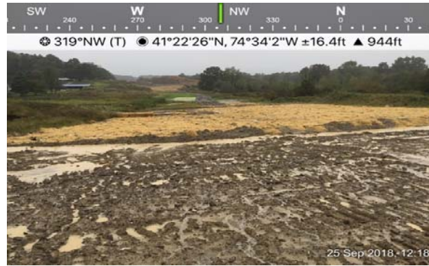
Photograph 2: STA 258+00 (Huguenot); Contractor has placed additional temporary seed and straw mulch.
