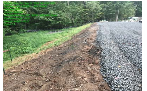
Photograph 8: Freshly contoured slope awaiting seed/much application (Ramapo).
