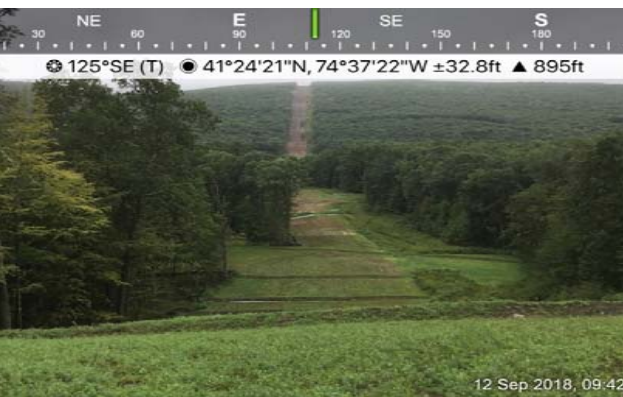
Photograph 4: STA 65+00 (Huguenot); Active restoration areas in various stages of vegetative growth.
