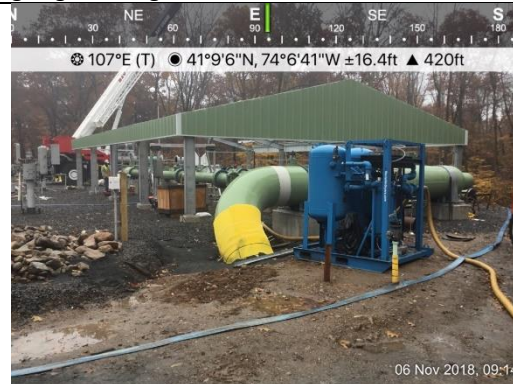
Photograph 8: (Ramapo) backfilling completed at north side of station
