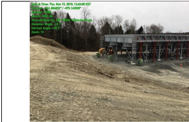
Photograph 5: (Hancock) preparing final grade for stabilization
