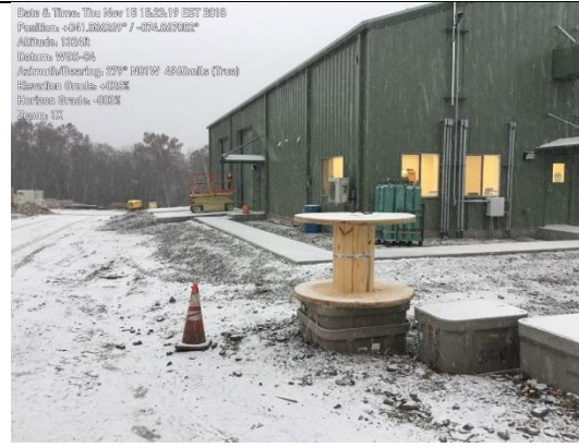
Photograph 2: (Highland) Office/warehouse building
