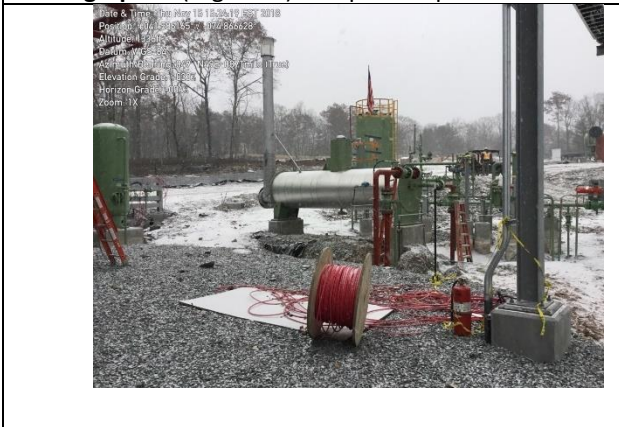
Photograph 3: (Highland) Auxiliary building pad
