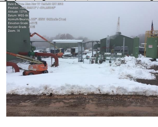
Photograph 4: (Highland) Compressor, Auxiliary and warehouse buildings
