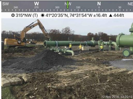
Photograph 7: (Huguenot) final restoration work for West Town facility
