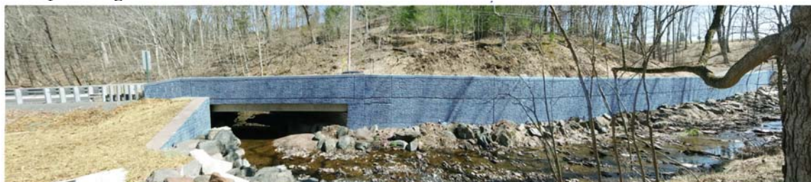
Cafferty Road Bridge as built
