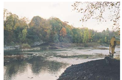
The site of the former Felix Dam.
