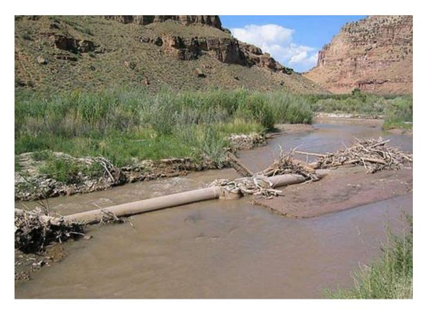
Photo from Fogg and Hadley (2007) of an exposed pipeline crossing an unnamed western US river. Here, lateral migration of a stream channel during high water excavated a section of pipeline under a floodplain that was several feet shallower than at the original stream crossing.
