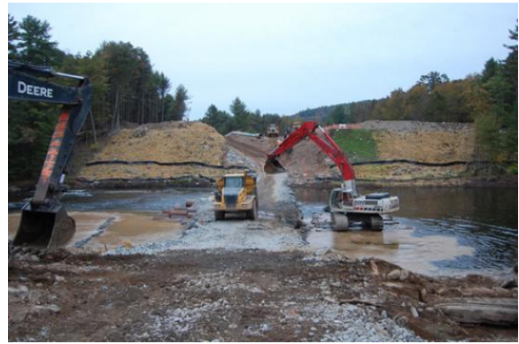
Figure 3: Picture of wet ditch crossing of the Lackawaxan West Branch River .
