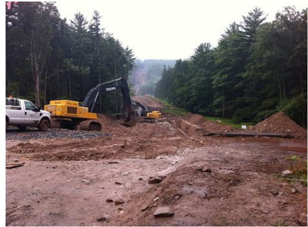
Figure 6: Picture of a natural gas pipeline construction in Pike County, Pennsylvania.
