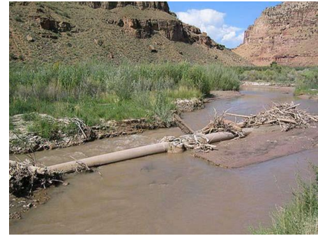
Figure 4: Picture of an exposed pipeline crossing an unnamed western US river.
