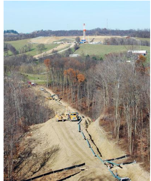
Figure 2: Picture of a well-pad and gathering line located in Amwel Township, Pennsylvania
