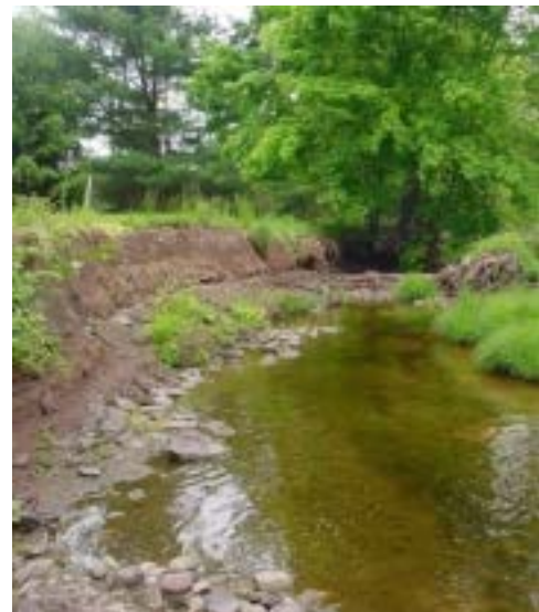
VALLEY CREEK, CHESTER COUNTY, DRN ASSISTED OPEN LAND CONSERVANCY AND RESTORED THIS STREAM REACH WHICH HAD BEEN DEVASTATED BY EROSION.
