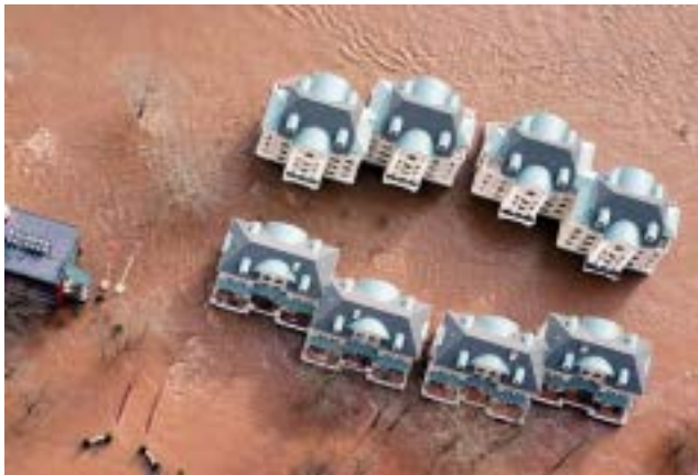
NEW HOPE, PA CONDOMINIUMS INUNDATED DURING THE JUNE 2006 FLOOD. THESE RESIDENCES WERE BUILT BETWEEN THE DELAWARE CANAL AND RIVER, IN A FRAGILE ENVIRONMENT SURROUNDED BY WATER WITH NO RIPARIAN BUFFERS OR PROTECTION FROM OR FOR THE RIVER.
