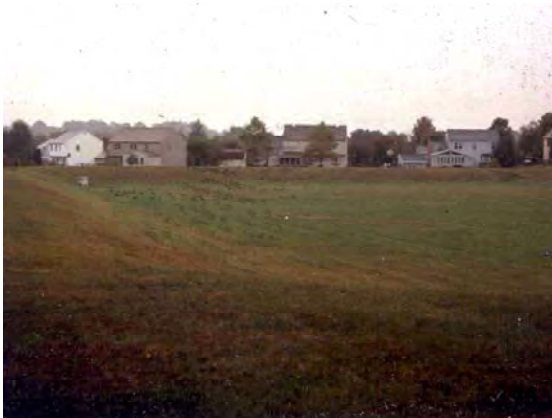
Conventional detention basin
