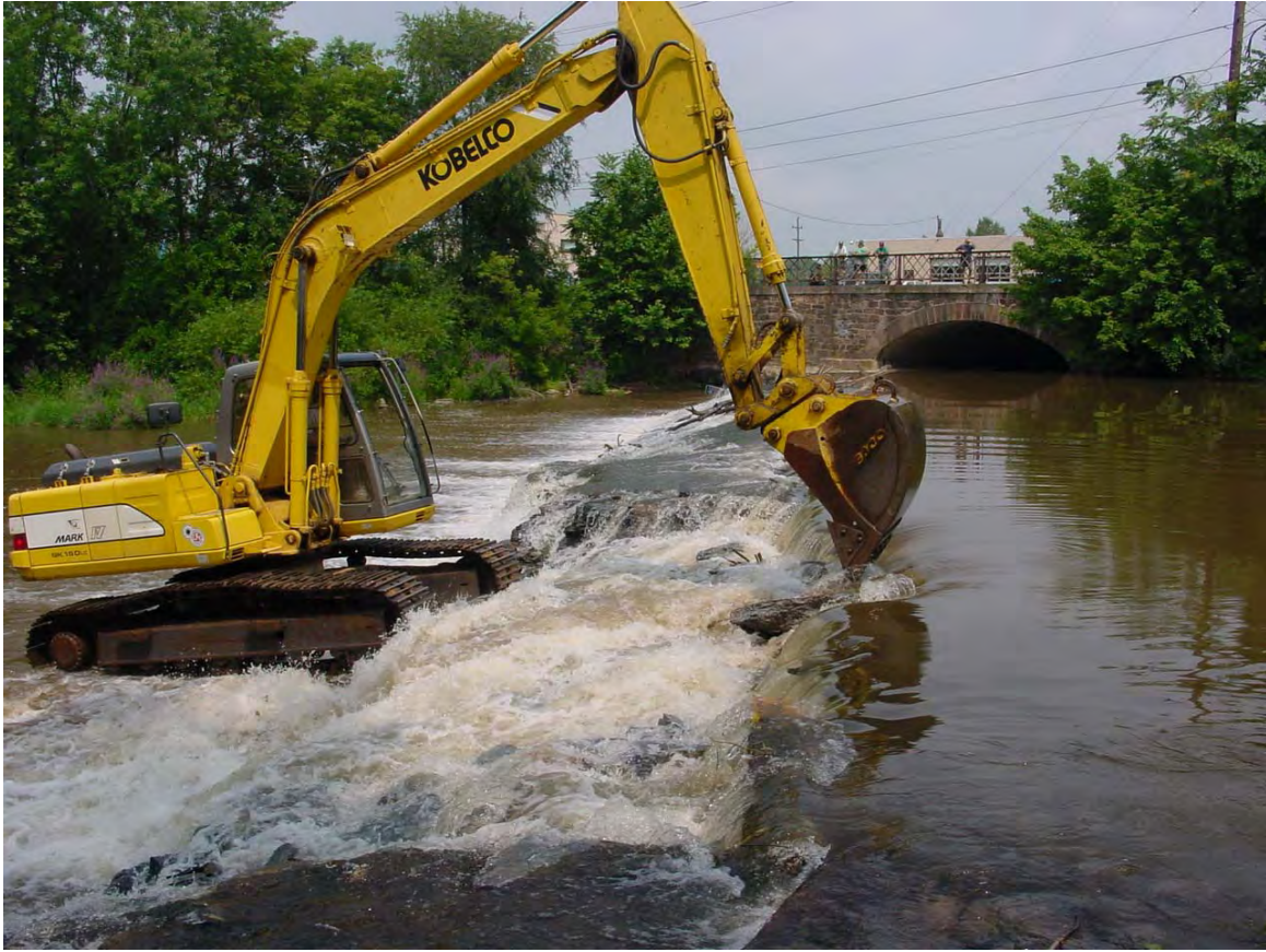
Removal of orphan dam on Manatawny Creek, Pottstown, PA.
