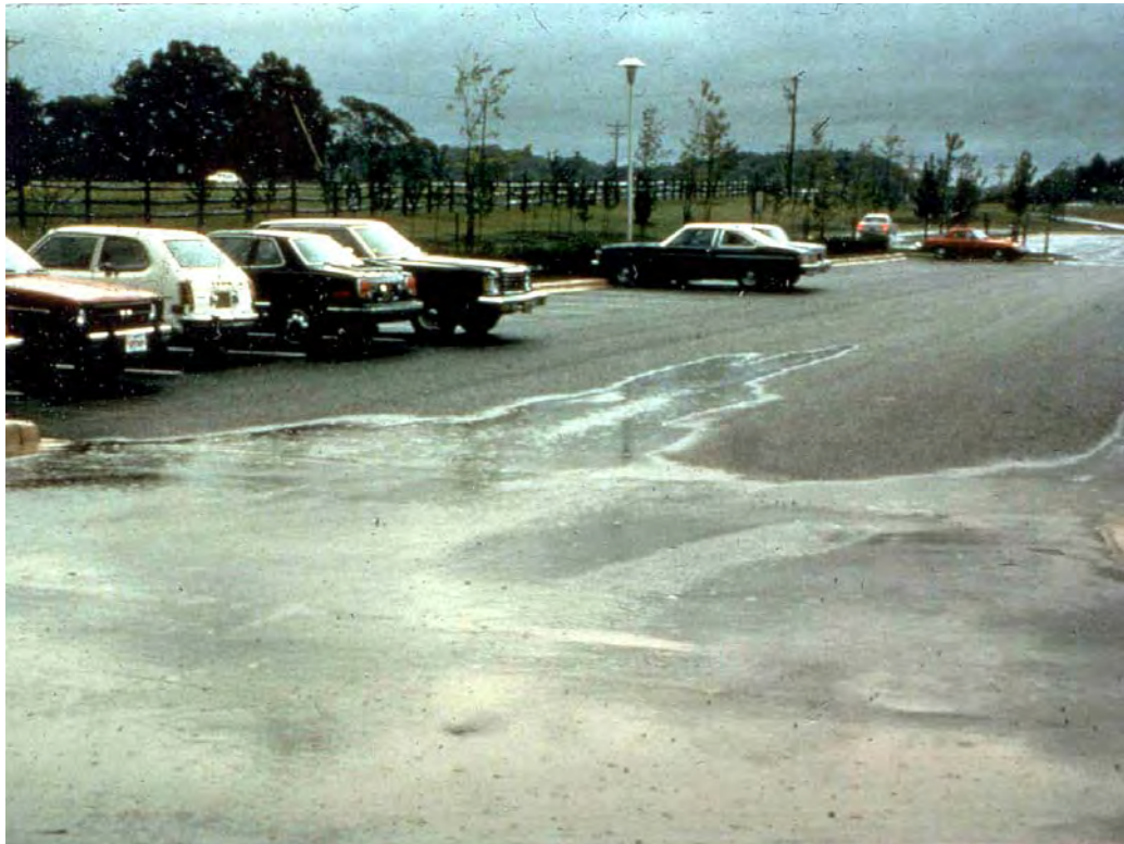
Left: Porous paving parking lot with recharge bed infiltrating stormwater from hurricane.
