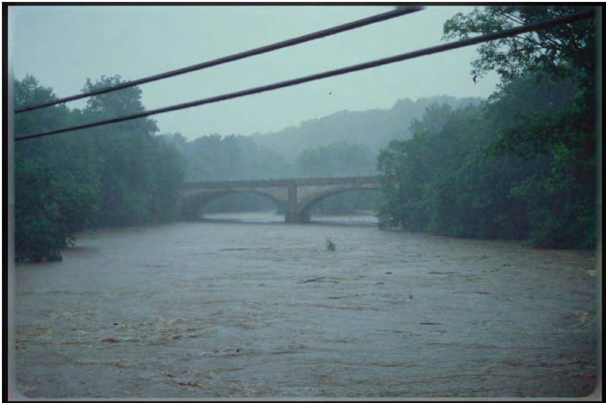
Flooding of the Neshaminy Creek during Hurricane Floyd
