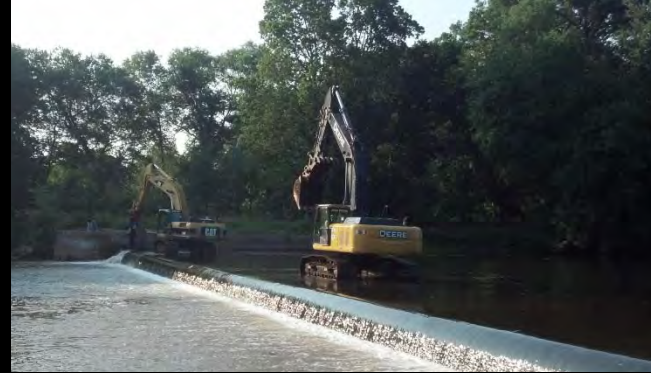
Roberts Street Dam, Raritan River, NJ
