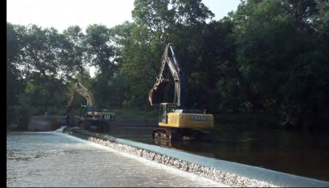
Roberts Street Dam, Raritan River, NJ
