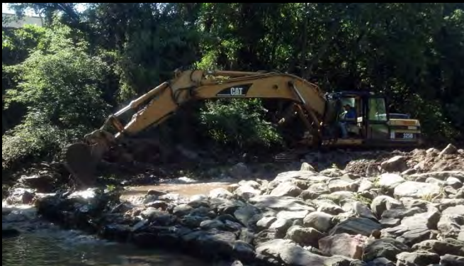
Kent Park Dam, Darby Creek, PA
