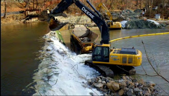
Simkins Dam, Patapsco River, MD
